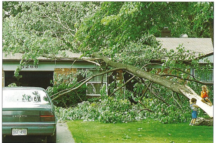
Figure 2. This damage was due to poor tree structure. Cabling would have minimized or avoided the damage.
